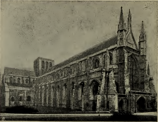
FROM NORTH WEST.
